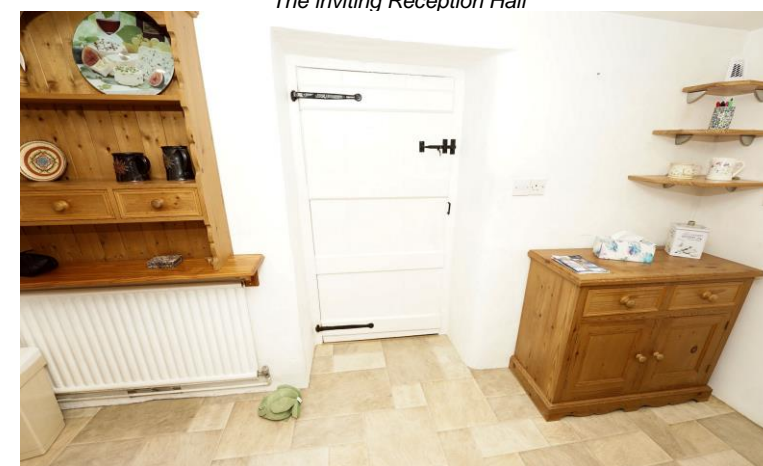
Period plank doors with strap hinges and Norfolk latches.
